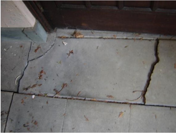
Damage in the entrance threshold
