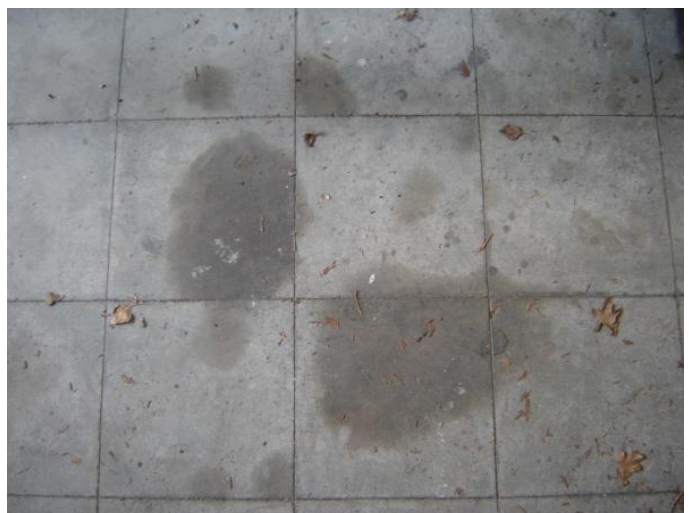
Oil stains on the concrete tiled floor
