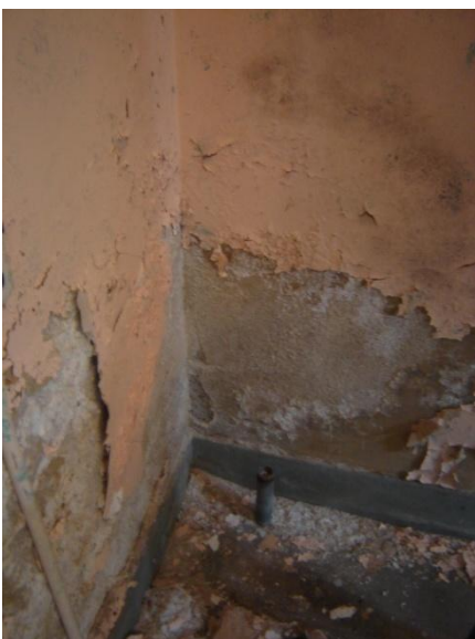
Corroded southwest wall
