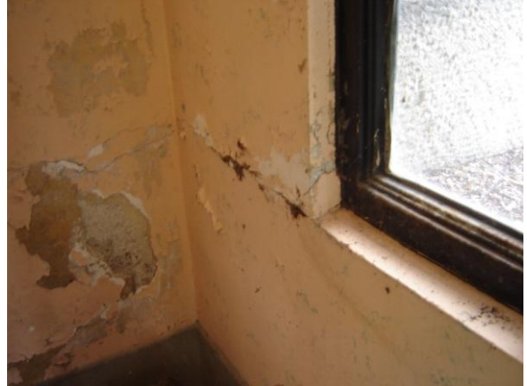
Damaged paint and plaster northwest corner
