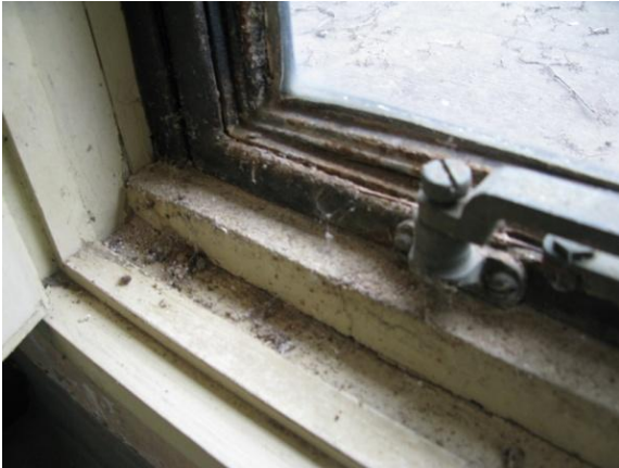
Rust damage in the north window hardware
